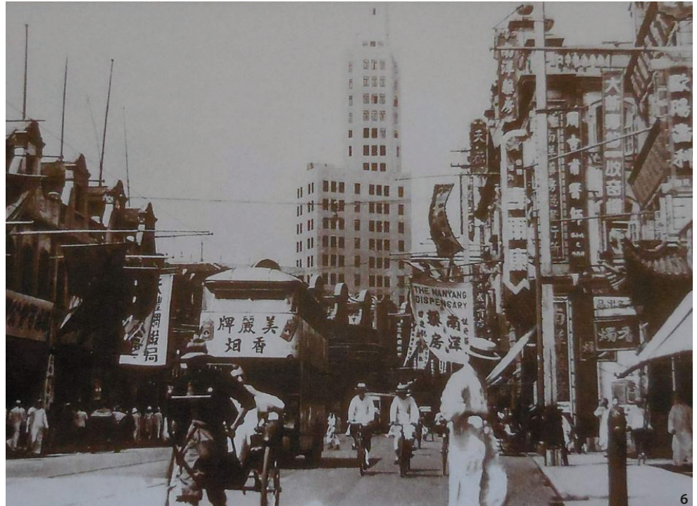
Figure 6 Wing On Department Store, Art Deco Tower, architects Elliot Hazard and Edward Phillips (Source: Peter Hack on abc.net.au).
