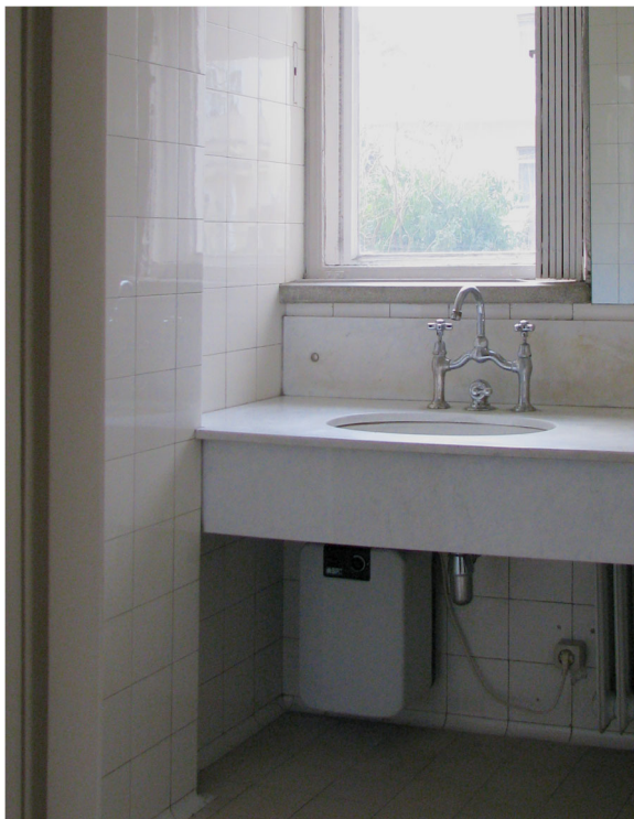
Fig. 23 Josef Frank and Oskar Wlach, Villa Beer in Vienna-Hietzing (1930), ground floor, entrance space of the toilet with largely preserved furnishings in finely graduated bright shades: carefully laid yellowish floor tiles and whitish yellow wall tiles (crimp joints), the washbasin with bright Carrara marble and original fixture (Source: Ivo Hammer 2017)
