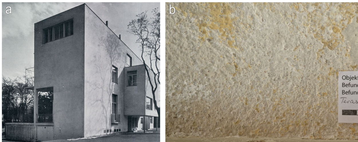
Fig. 17 Josef Frank and Oskar Wlach, House Beer in Vienna-Hietzing, 1930. a: from northwest. On the northern façade, the traces of the facture can be seen: scaffolding borders, irregularities [Source: Julius Scherb, Vienna 1931]. b: roof terrace, sunbathing niche, ceiling, original façade surface with remnants of four later overcoats and salt efflorescence, yellowish lime wash pigmented with fine silicates on grated lime plaster (Source: HABEAS 2017)
