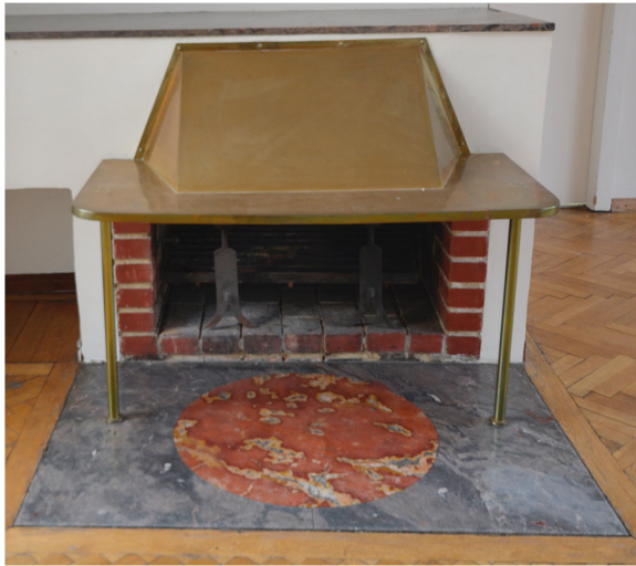
Fig. 25 Josef Frank and Oskar Wlach, Villa Beer in Vienna-Hietzing (1930), living room, fireplace with polished slabs of reddish limestone ('onyx' marble), crinoid limestone and brass chimney (Source: Ivo Hammer 2017)
