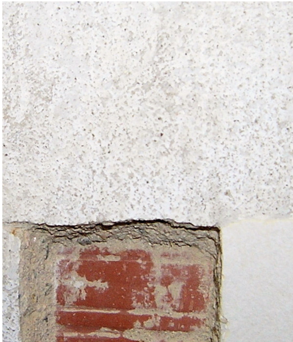
Fig. 12 Pavel Janák, Brno, fair grounds, pavilion of the Prague School of Applied Arts, 1928, original facade plaster: the surface rubbed, with thin, bright fresco-lime wash, similar to the later one at the house Tugendhat (Source: study work HAWK / Hildesheim, Ivo Hammer, Silke Heinemann and Jan G. Menath, 2005)
