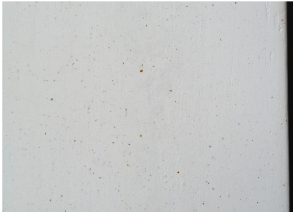
Fig. 22 Ludwig Mies van der Rohe and Lilly Reich, House Tugendhat, Brno, 1930, bedroom Fritz Tugendhat, 2011 reconstructed 'stucco lustro' (preservation by covering) (Source: Ivo Hammer 2013)
