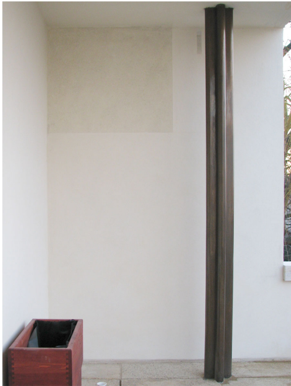
Fig. 8 Ludwig Mies van der Rohe and Lilly Reich, Tugendhat House, Brno (1930), upper terrace, view to the southeast: ‘Archaeological window’ (campione), which shows the original facade surface. The lime wash of the remaining façade surface, re-established according to the historic tradition of repair and renewal, is kept lighter because it darkens as it ages (Source: Ivo Hammer 2012)
