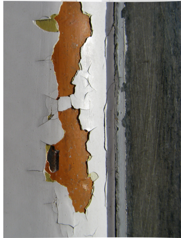
Fig. 18 Josef Frank and Oskar Wlach, Villa Beer in Vienna-Hietzing (1930), west facade, main entrance, metal door frame, detail with remains of the original 'Japanese red' paint (Source: Ivo Hammer 2017)
