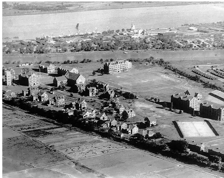
Fig. 13 Shanghai College under construction (Source: Archives of USST)
