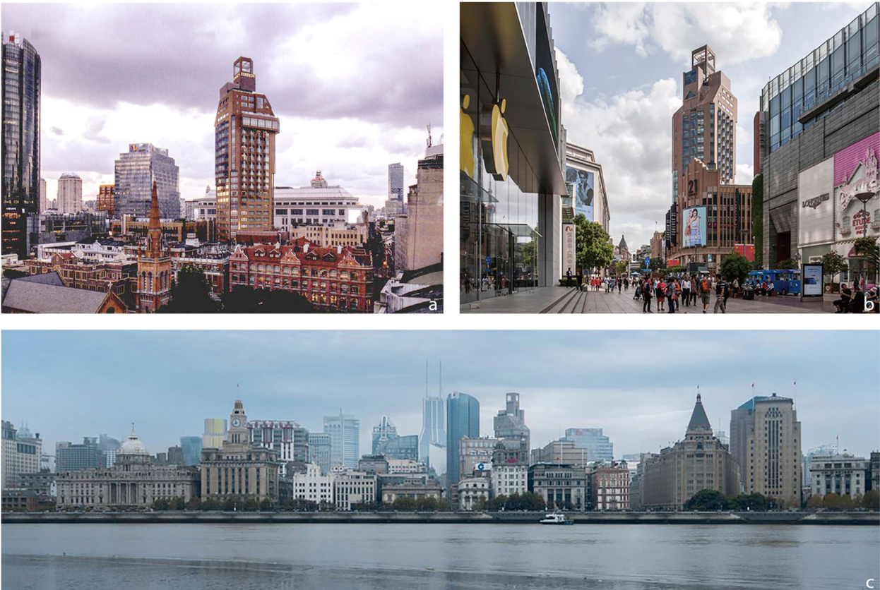
Fig. 13 SECEP Building in its urban context after renovation (2018) (Sources: a, b Fan 2018; c Peng and Dong 2018)
