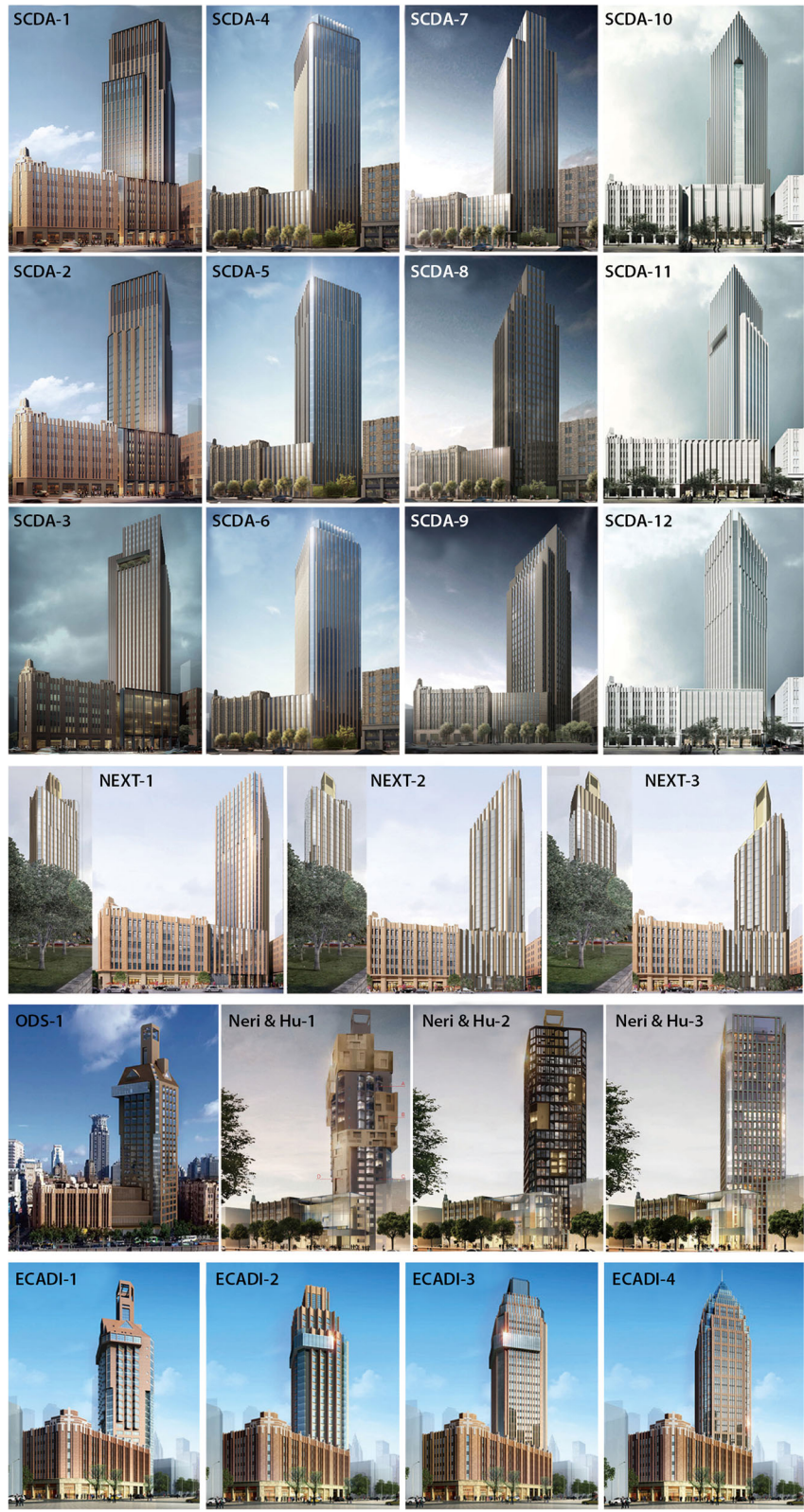
Fig. 10 Renovation proposals for the SECEP Building (Source: Images provided by ECADI)
