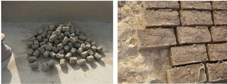
**Fig. 9** Left: Old style mud bricks in Djenné (Djenné Ferey). Right: and new type of bricks (toubabou ferey). August 2009 (Source: the author)
