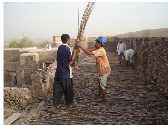
Fig. 5 Zabid, traditional roofing with brushwood (Source: the author)
