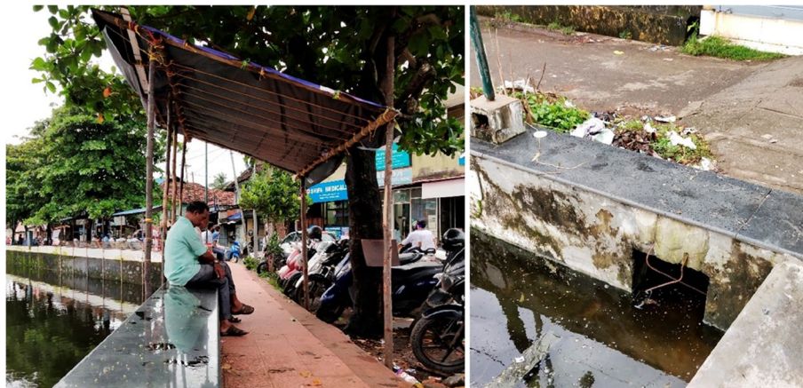
Fig. 6 Temporary sheltered seating and water drainage (before revitalisation). (Source: the authors)
