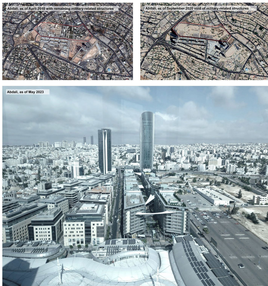
Fig. 8 The Abdali 'State Zone', as it appears in contemporary times, with global high-rise structures to represent neo-liberal urbanism and open lots in the place of the old military sector (Source: maps were modified from Google Earth Pro; photograph captured by the author on May 20th, 2023)
