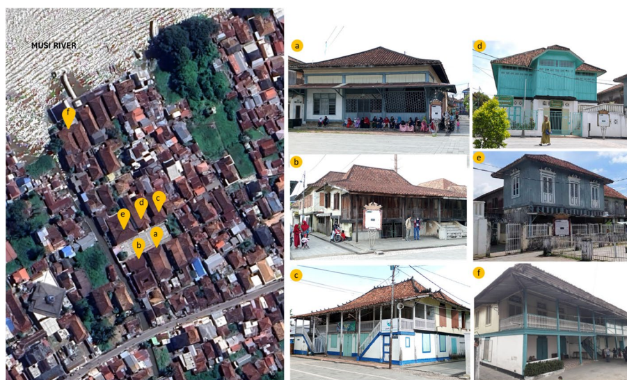
Fig. 2 The observed traditional houses in the Arabic Kampung Al Munawwar 13 Ulu, South Sumatera, Indonesia, 2023 (Source: Google Maps and the authors)
