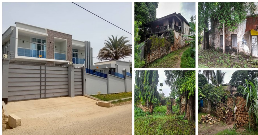
Fig. 7 New buildings constructed in the historic town, while some of the old buildings are in a poor state of conservation (Source: the authors)
