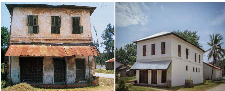
Fig. 4 Pictures showing the Pangarithi building before and after rehabilitation (Source: UZIKWASA)
